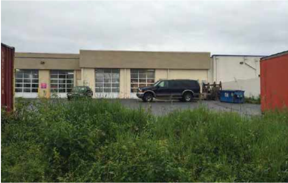
Target Property 3 - Photo 04 - Overview of Quick Lube from West
