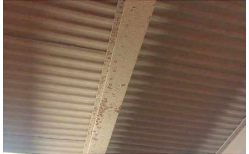
Photo 10 - Lead-Positive Ceiling (Boxing Studio)
