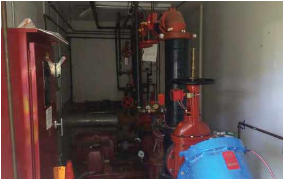
Photo 07 - Sprinkler System
