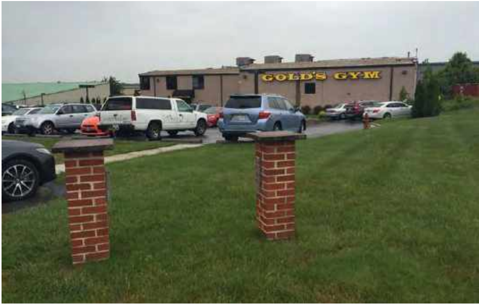
Photo 01 - Overview of Site
