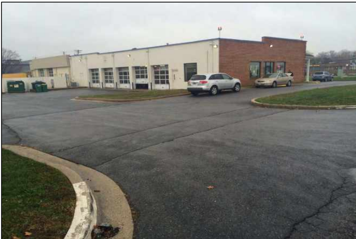
Figure 4: Parcel 29, facing northeast toward Woodfield Road
