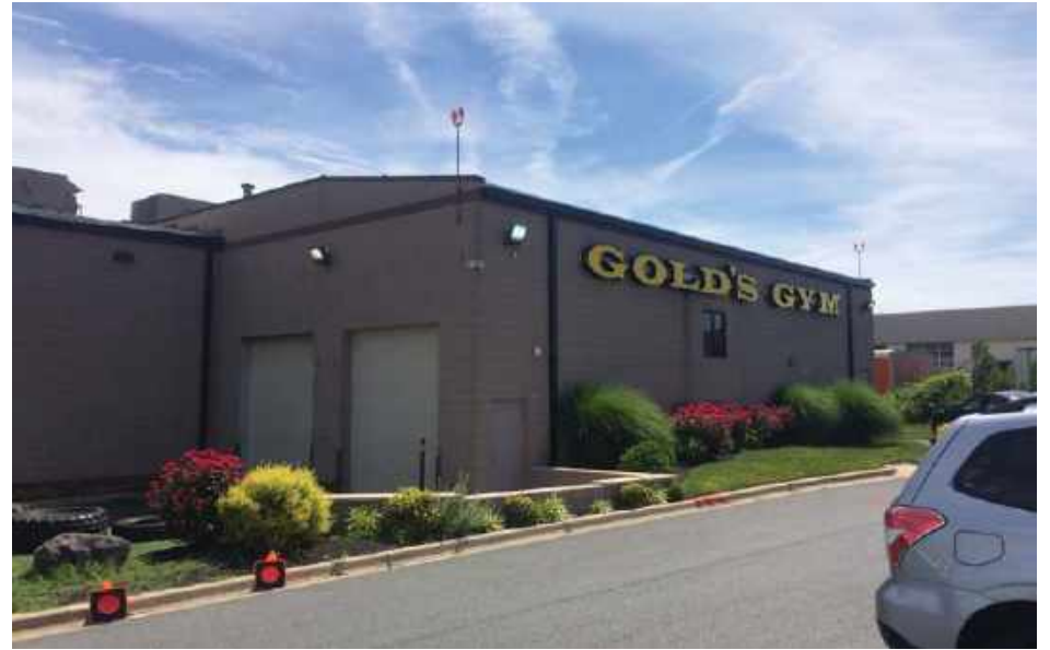
Photo 02 - Front of Building
