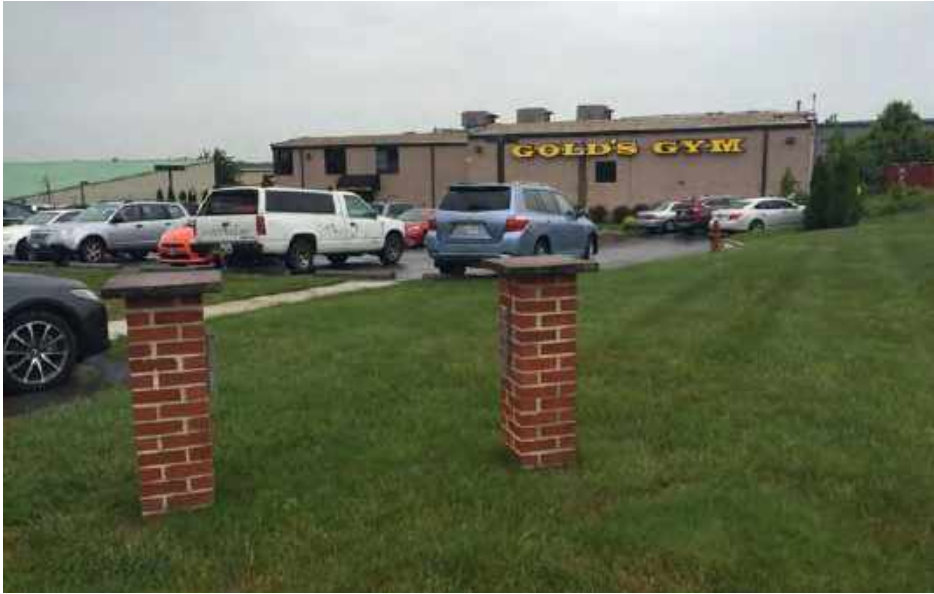
Photo 01 - Overview of Site
