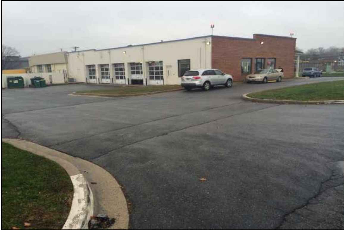
Figure 4: Parcel 29, facing northeast toward Woodfield Road
