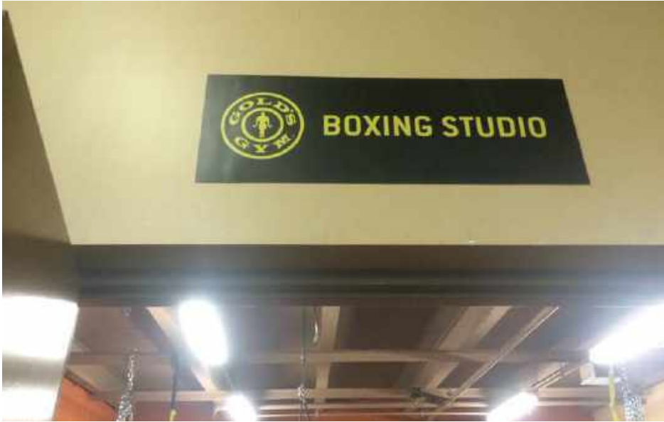
Photo 09 - Lead-Positive Ceiling (Boxing Studio)
